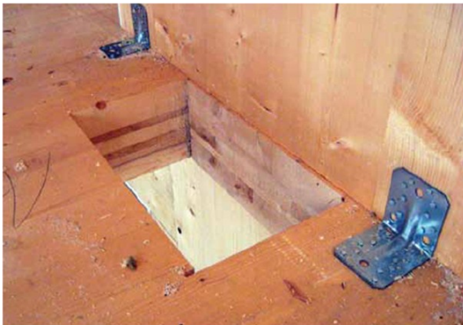
Figure 2. Metal bracket fastener system.
